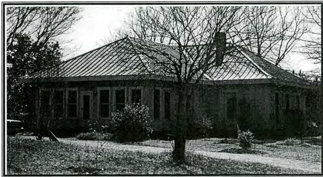
Figure 42 - Dodge Hunting Lodge Auxiliary Building
