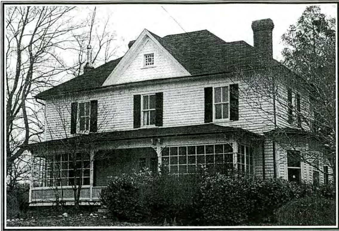
Figure 44 - Futrell-Mackay-Armstrong House (front elevation)
