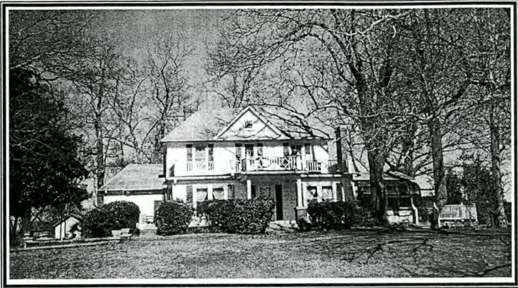
Figure 10 - L. W. Causey House
