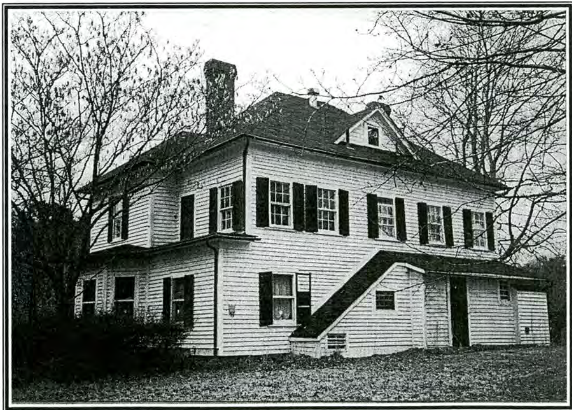
Figure 45 - Futrell-Mackay-Armstrong House (rear elevation)
