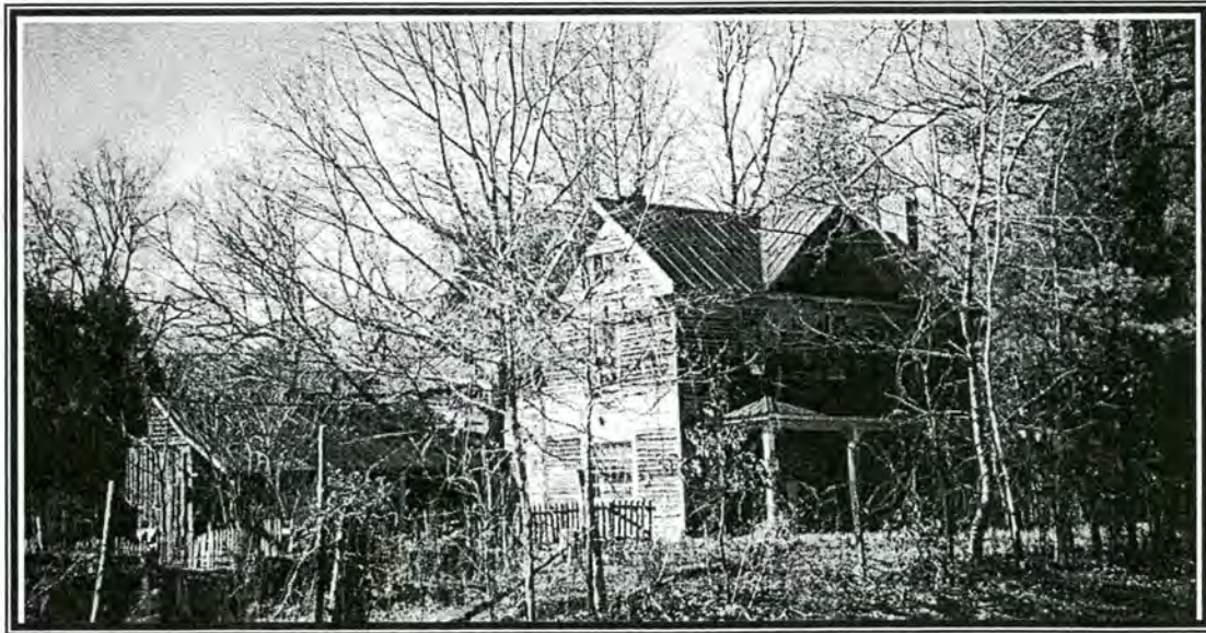
Figure 13 - Thomas Fentress House
