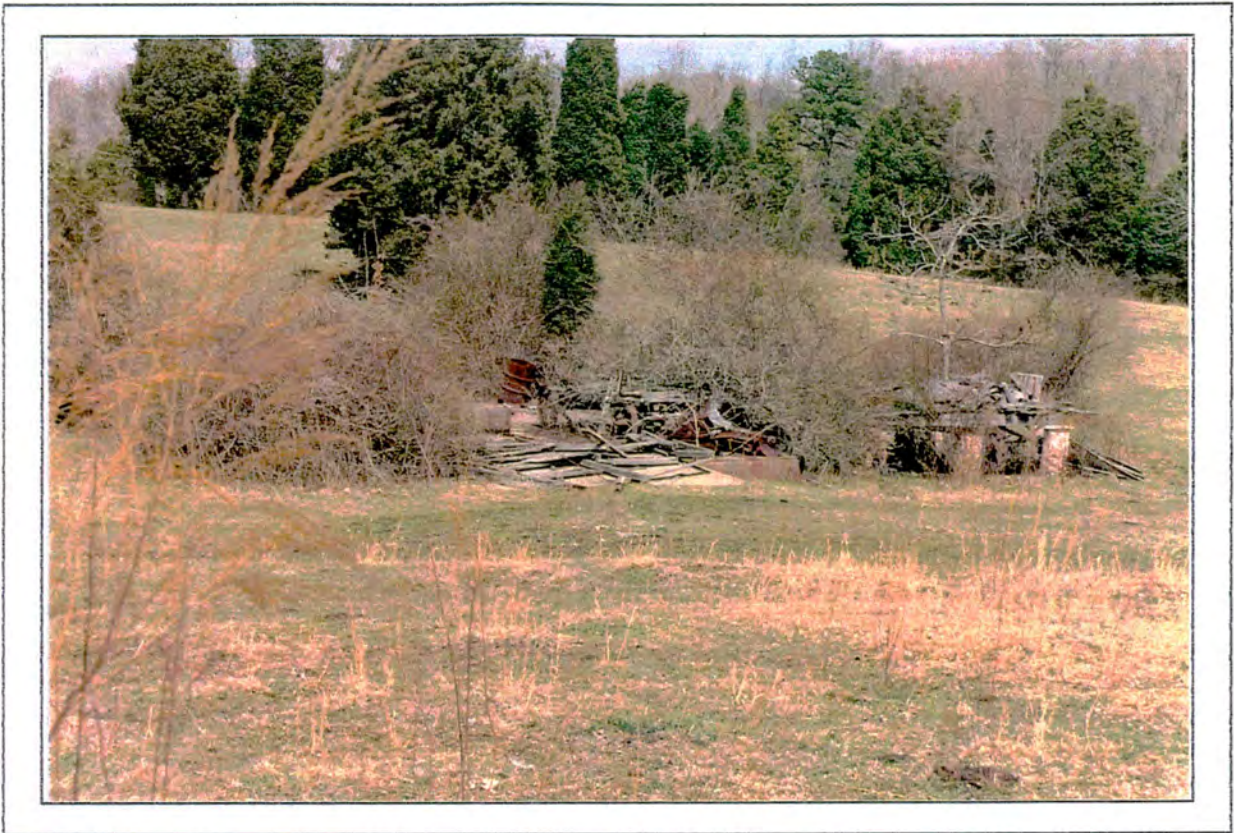
The Futrell-Mackay-Armstrong House Foudations of the Wagon House
