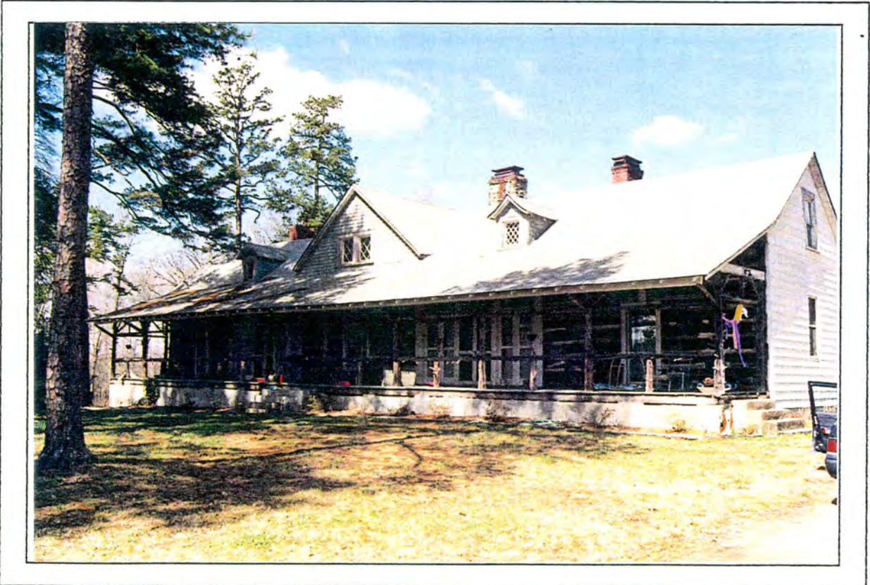
The Gould Lodge--Manager's House
