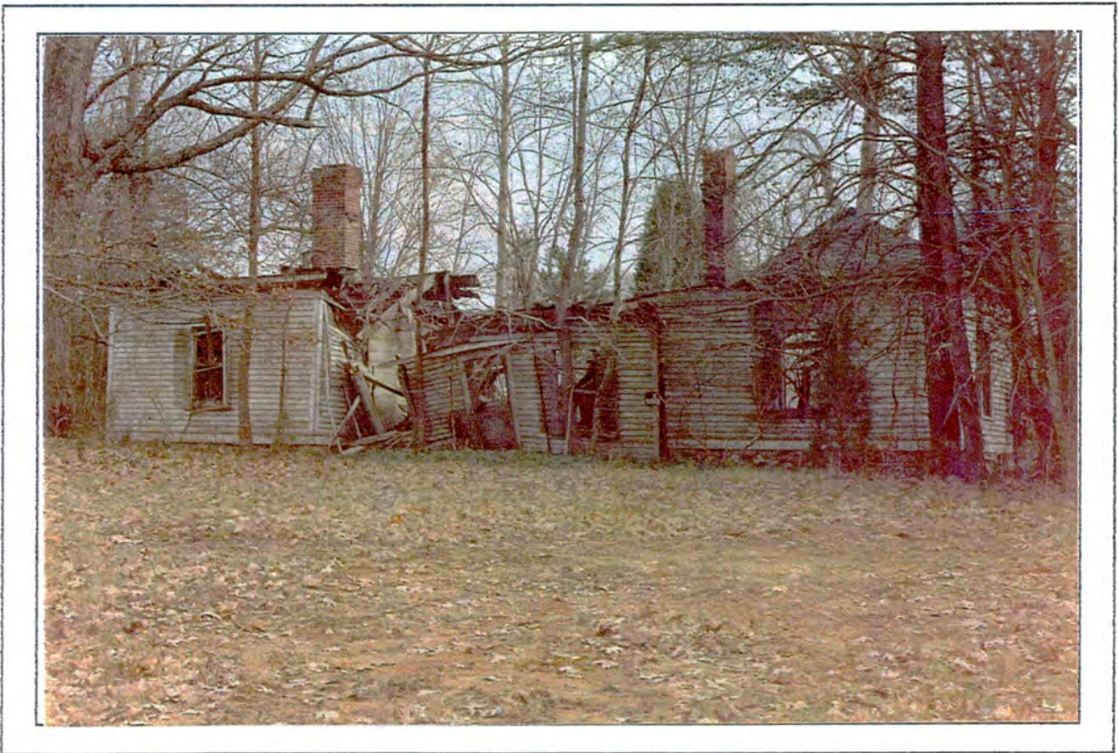
The Furtell-Mackay-Armstrong House Employee's Quarters (Building #10)
