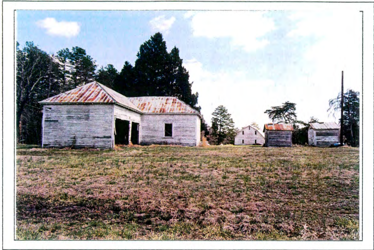
The Gould Lodge--Outbuildings and grounds
