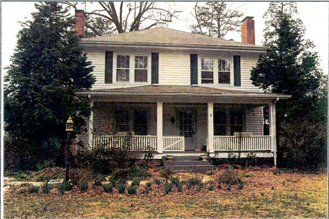
Climax Lodge--Manager's House
