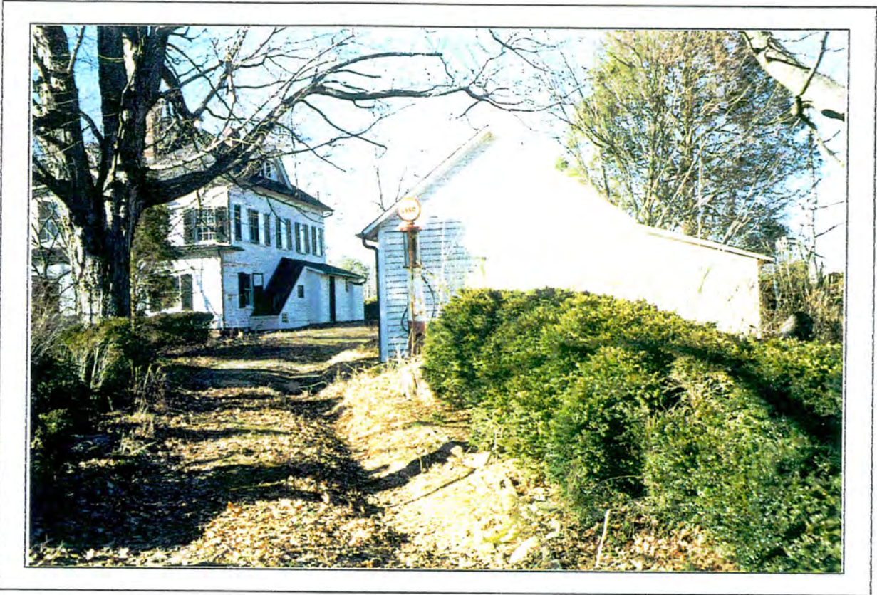
The Futrell-Mackay-Armstrong House--house, shed, and grounds
