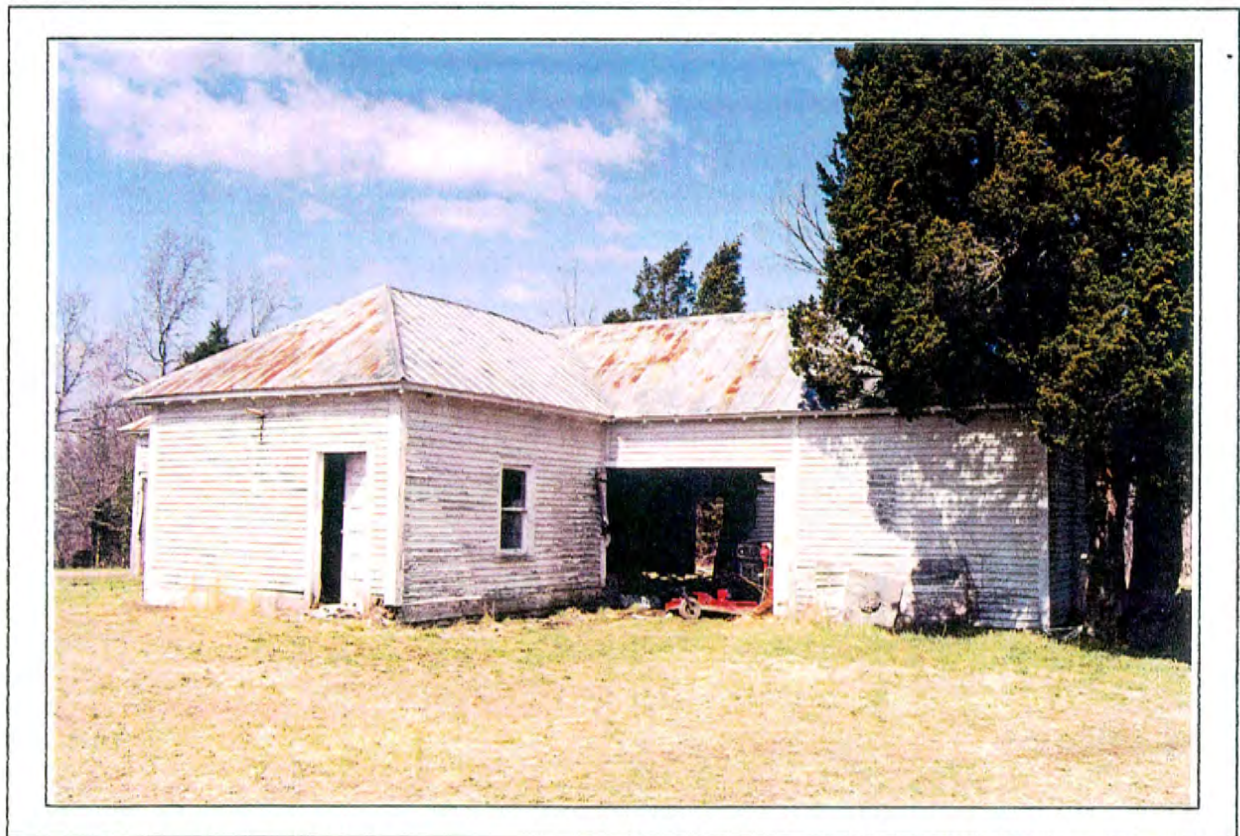
The Gould Lodge--Shed
