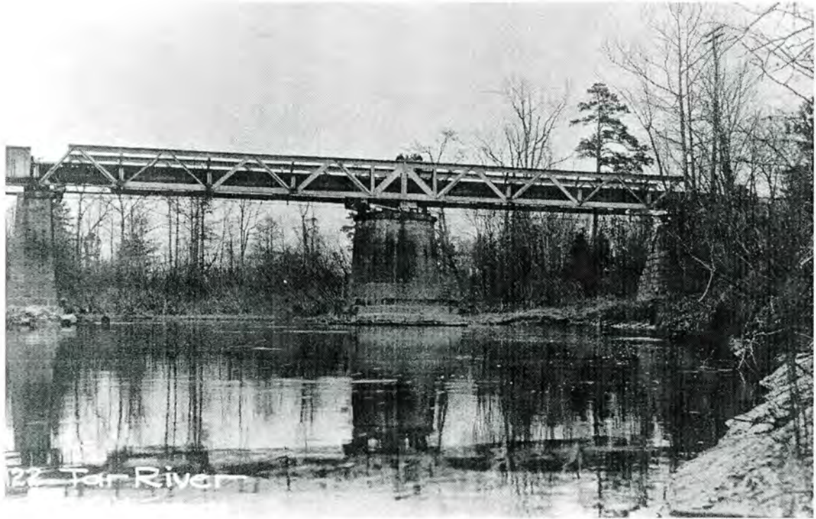
Figure 11. Looking north towards the swing span constructed between 1890 and 1913. Private Collection. The photograph is identified on its reverse as "Milepost AB 138.2, Tarboro to Kelford line" and dated to ca. 1910.
