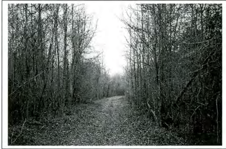
Figure 14. Railroad bed looking east from the bridge
