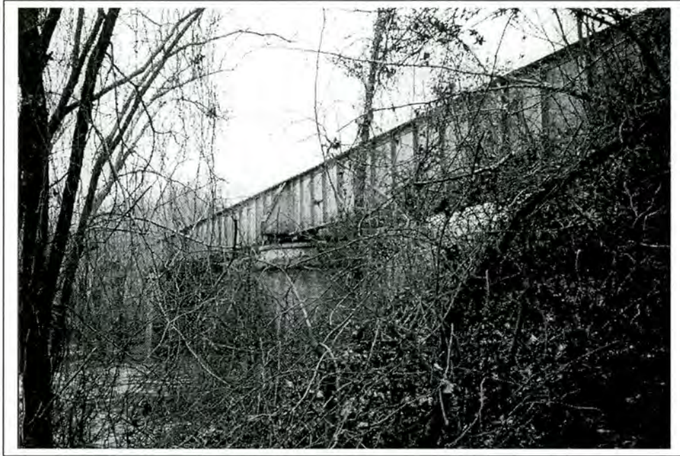
Figure 2. General view from the eastern bank of the Tar River.
