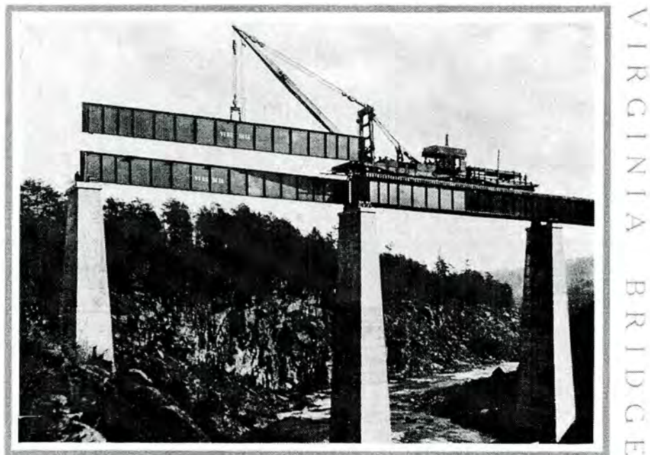
Figure 12. A deck plate girder railroad bridge under construction. The view appeared in an advertising brochure and shows a "derrick car" lowering into place a plate girder spanning 100 feet. From Virginia Bridge and Iron Company , 1915.
