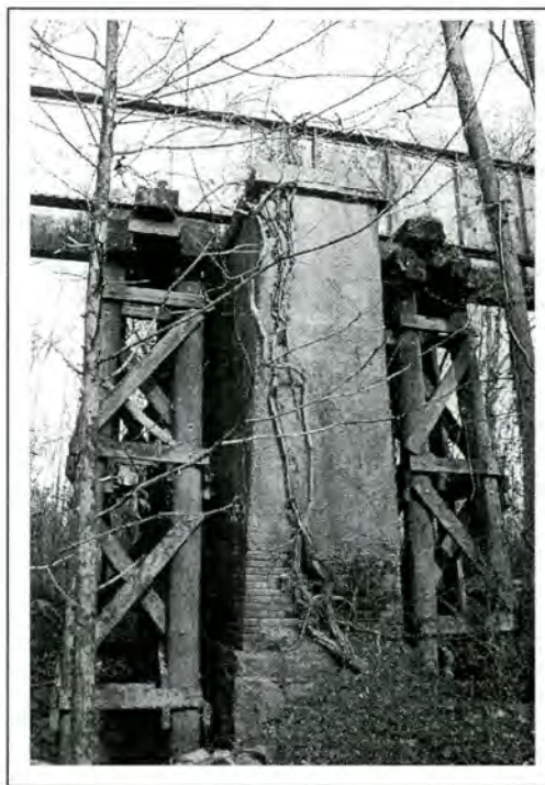
Figure 7. Pier with flanking bents at western end.
