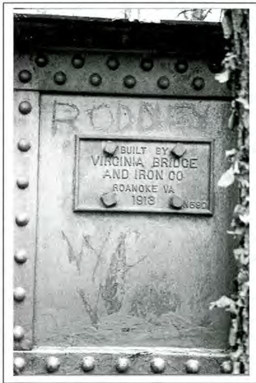
Figure 3. Manufacturer's identity plate. Interior south side, east end.
