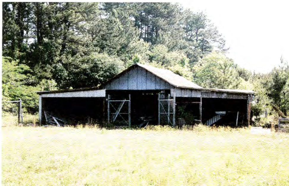
Figure 31. Property 2 - Landfill shed. The property has been determined not eligible for the National Register because it is neither historically nor architecturally significant. Photographed May 24, 2001.
