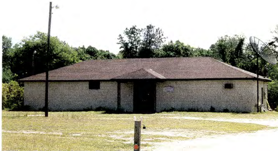
Figure 33. Property 4 - Panola Heights Club. The property has been determined not eligible for the National Register because it is neither historically nor architecturally significant. Photographed April 26, 2001.
