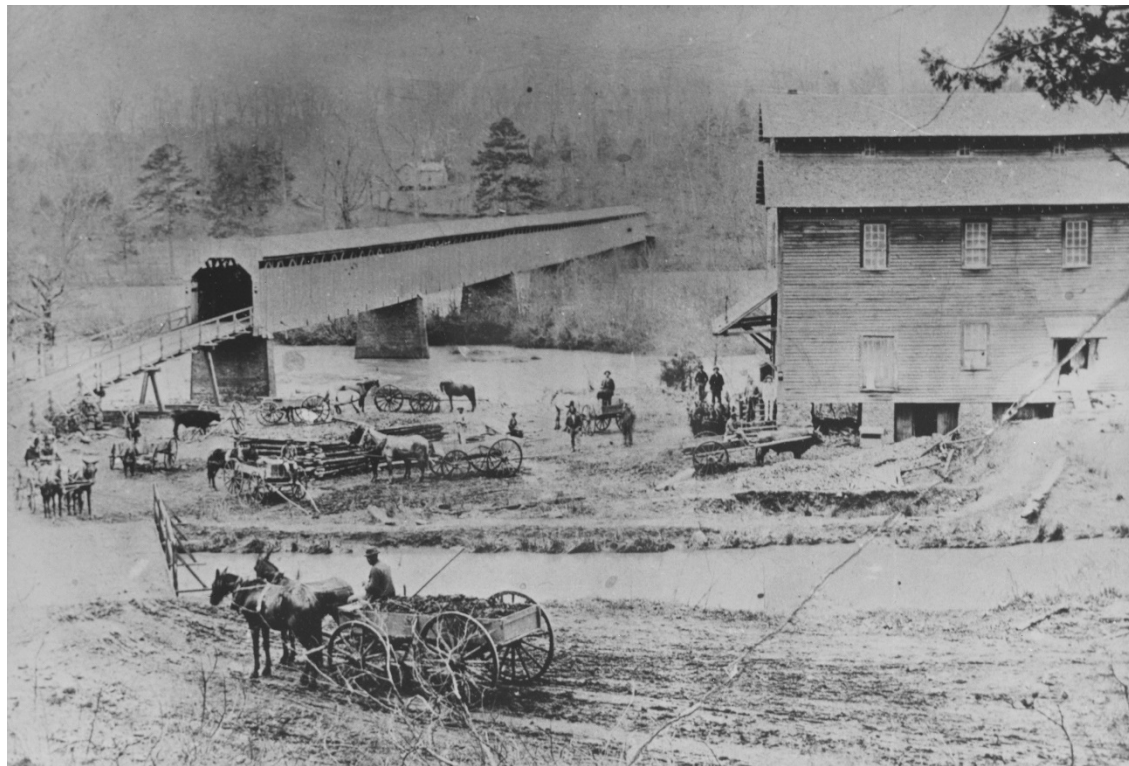
Figure 3 - Late 19th c. photo of covered bridge and mill at Bynum, looking west from the east bank.
