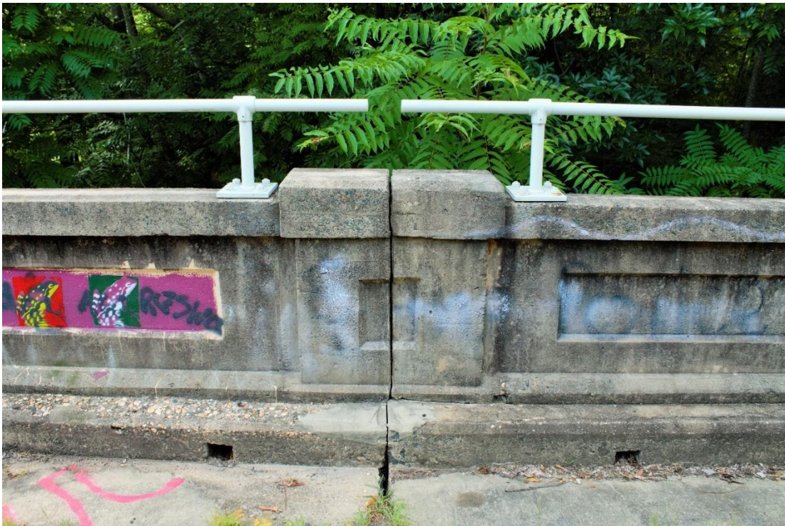
5. Detail of solid parapet and 1999 handrail at a joint between spans
