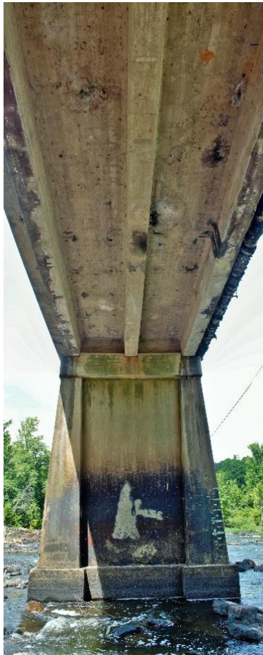
7. View from beneath bridge, showing pier, beams, and underside of decking
