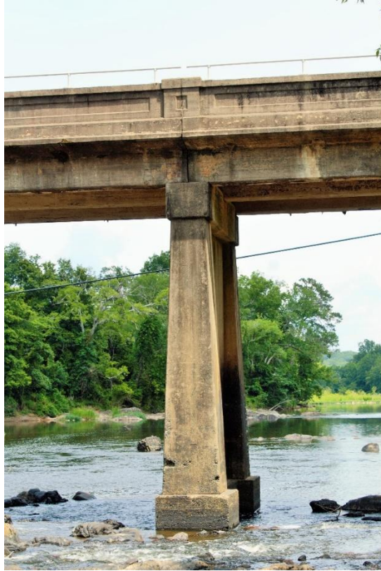
6. Sample pier and superstructure, from north
