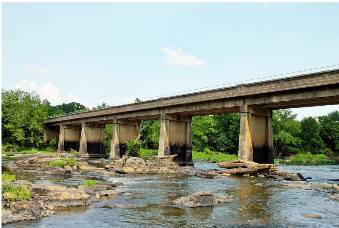
1. View from Haw River, looking southeast
