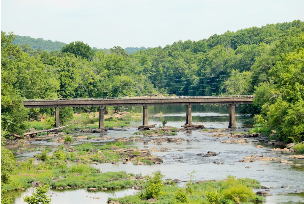
View of Bynum Bridge from US 15-501 bridge, looking south.
