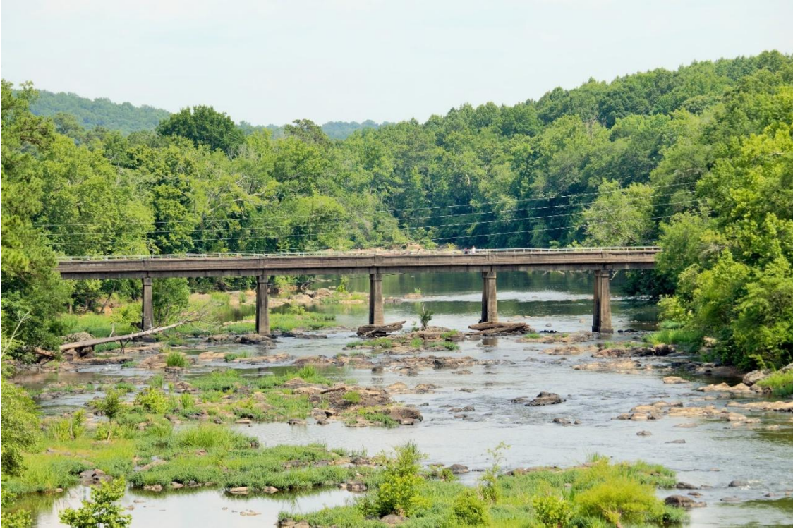
2. View from US 15-501 bridge, looking south
