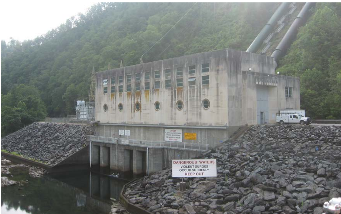
Powerhouse exterior, west elevation
