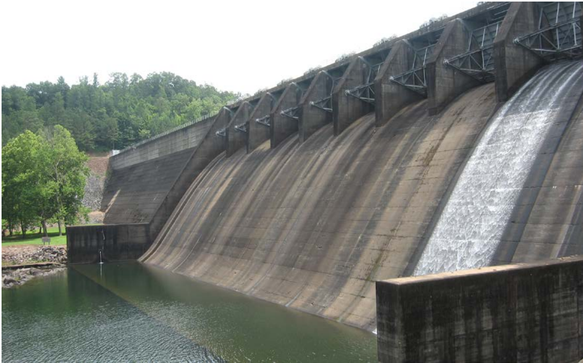
South side of Apalachia Dam
