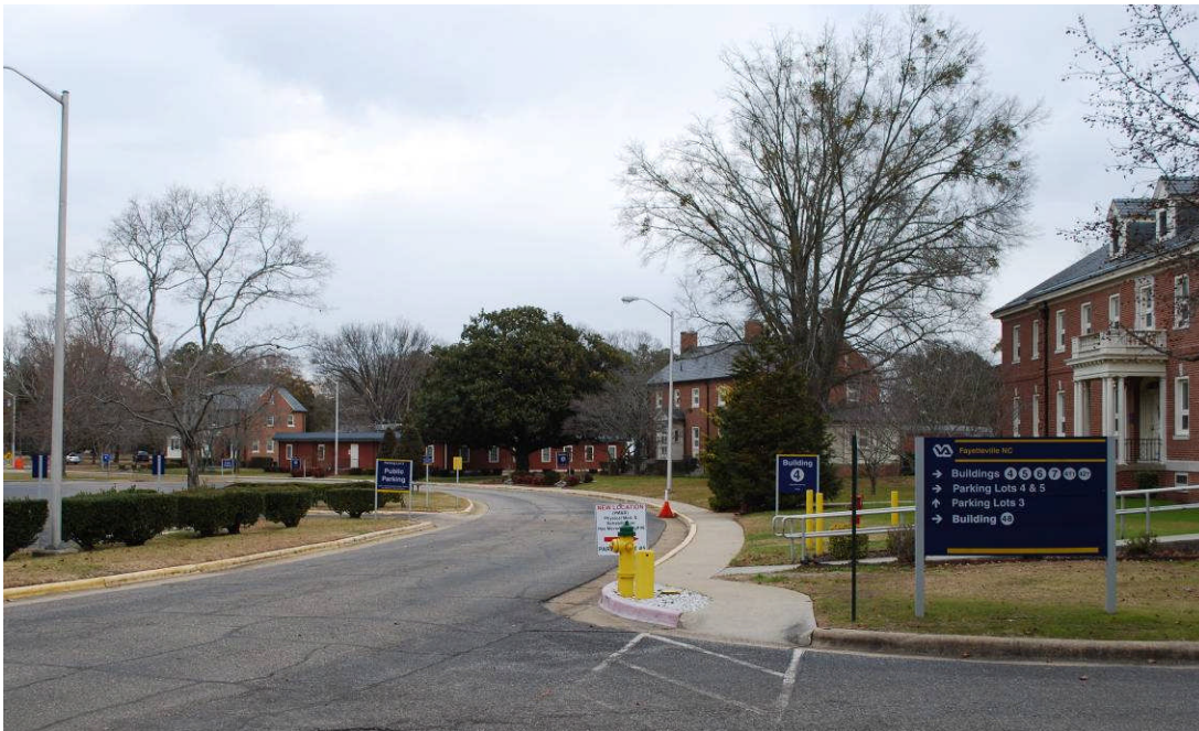
View north on Entrance Drive
