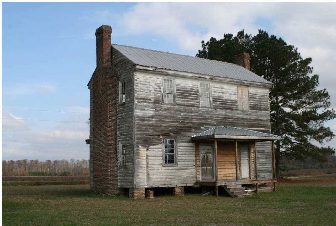
Side and rear view
