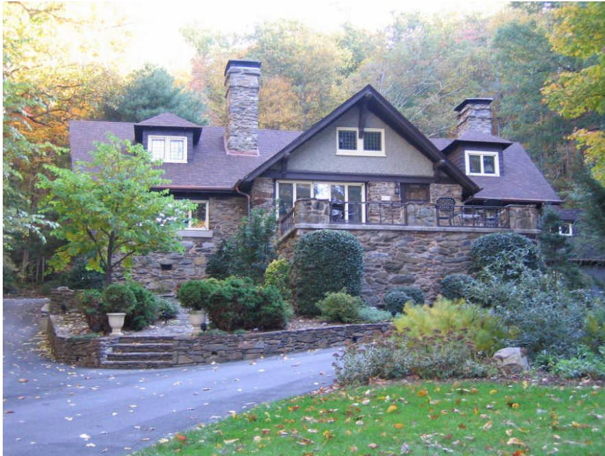
Overall view from street
