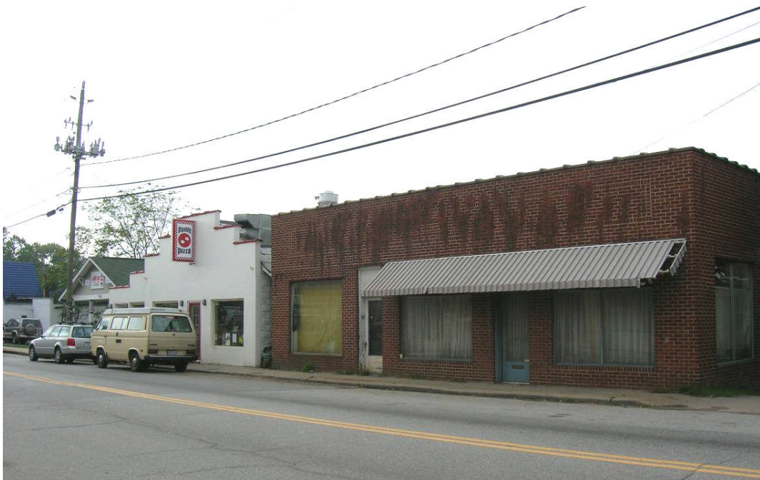
Haywood Road, south side, looking southeast
