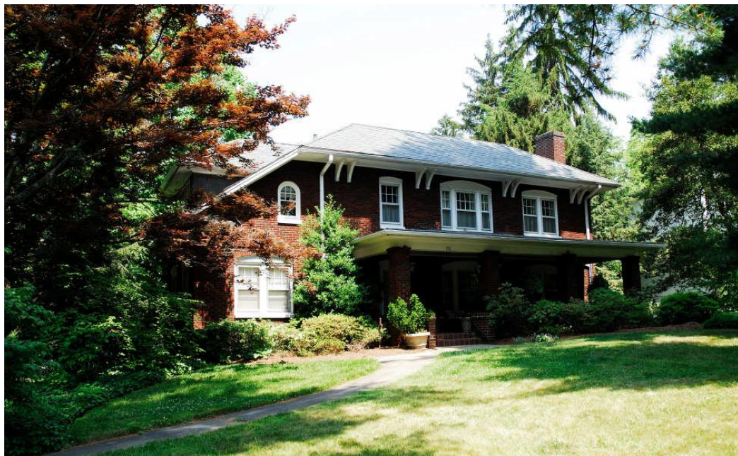
C. C. Willis House, 76 Macon Avenue
