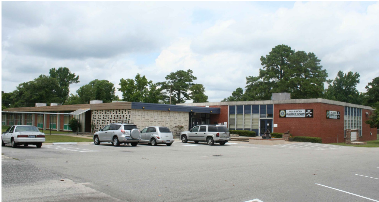
Front (southeast) and side (southwest) elevations of high school building, facing north
