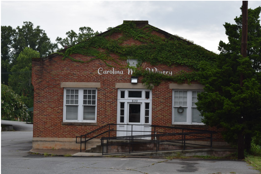
Façade, view east
