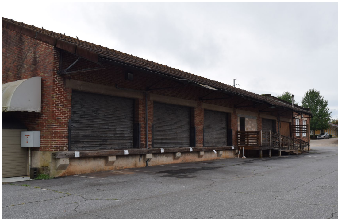
North elevation, view southwest
