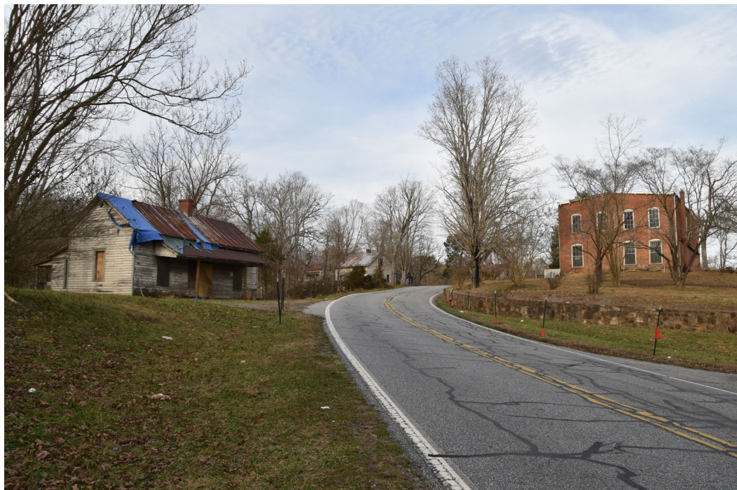
Henry River Road, view to northeast from north end of Henry River Bridge
