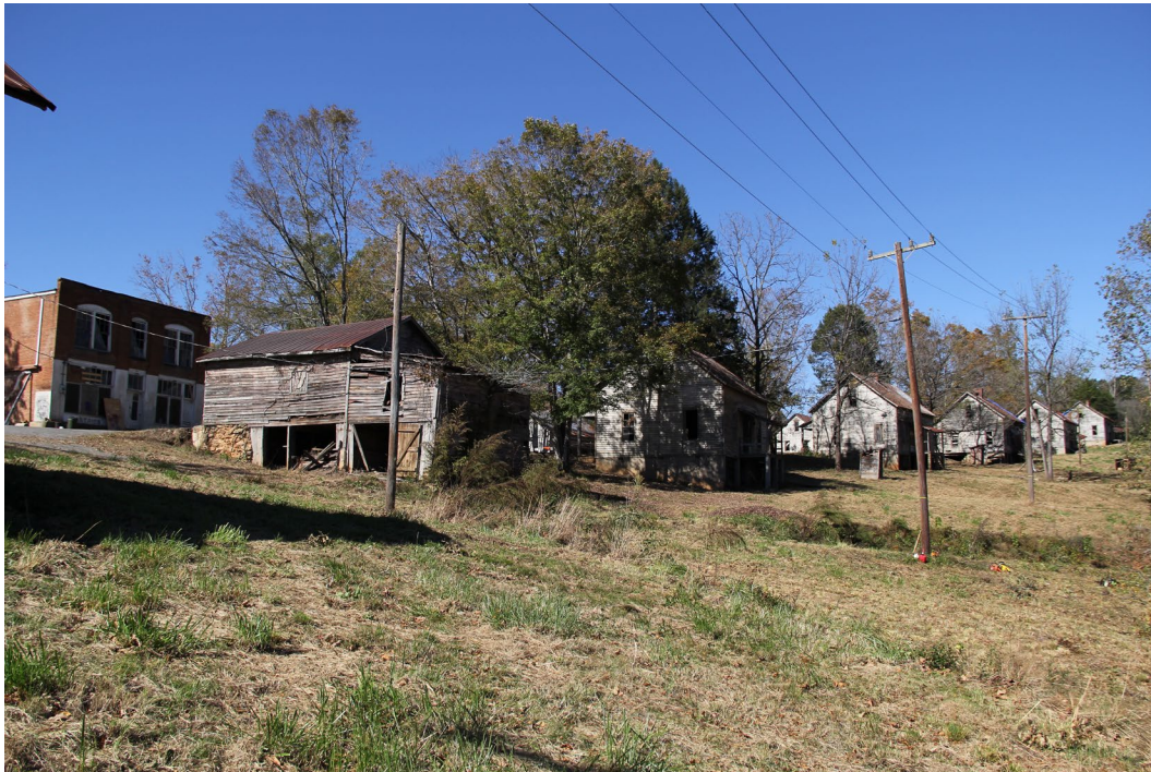
Mill houses, garage, and company store, overall view to northwest
