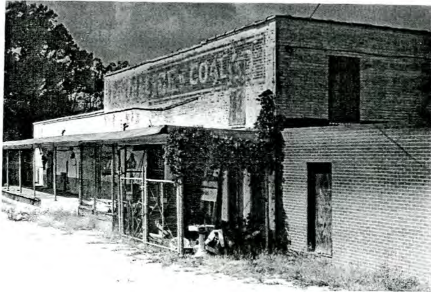
Plate 21. High Point Ice and Coal Company Building, Looking West.
