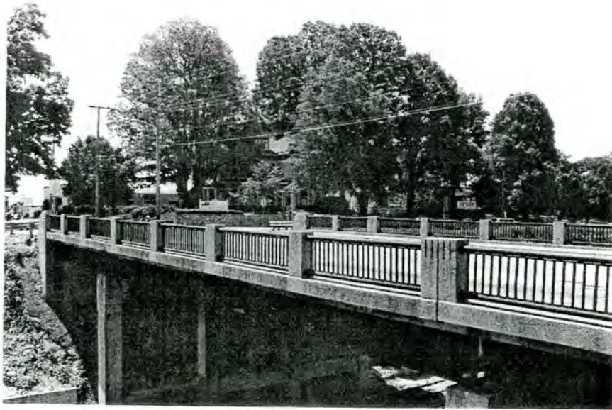
Plate 7. West High Street Residential Area, Looking South from Bridge No. 386.
