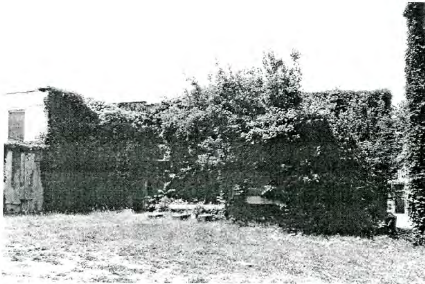
Plate 22. High Point Ice and Coal Company Building, Rear Wing, Looking West.
