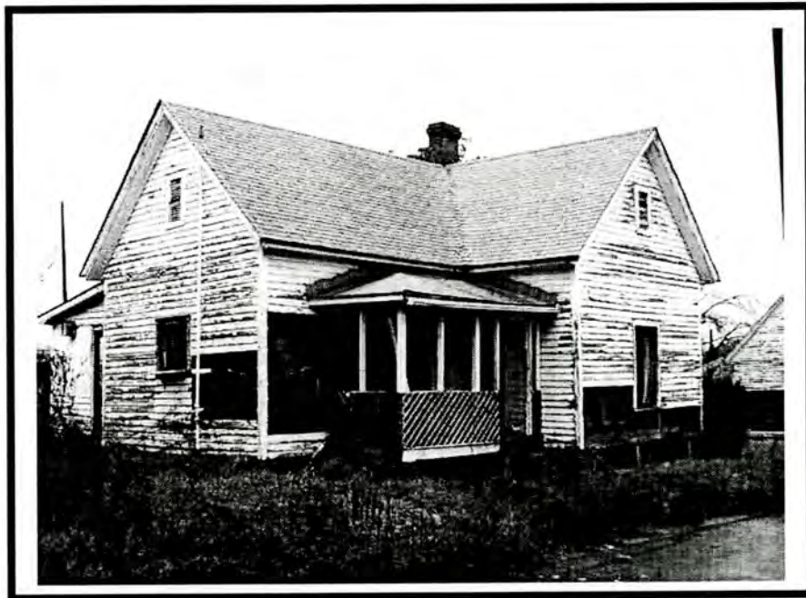
Figure 23 – Allen Street Mill Houses, House No. 10
