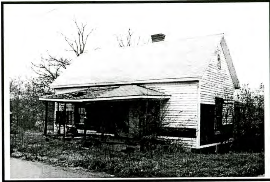
Figure 20 - Allen Street Mill Houses, House No. 7
