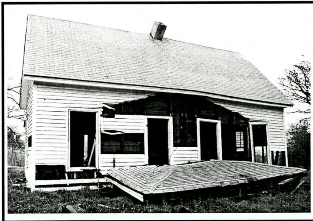
Figure 17 – Allen Street Mill Houses, House No. 4
