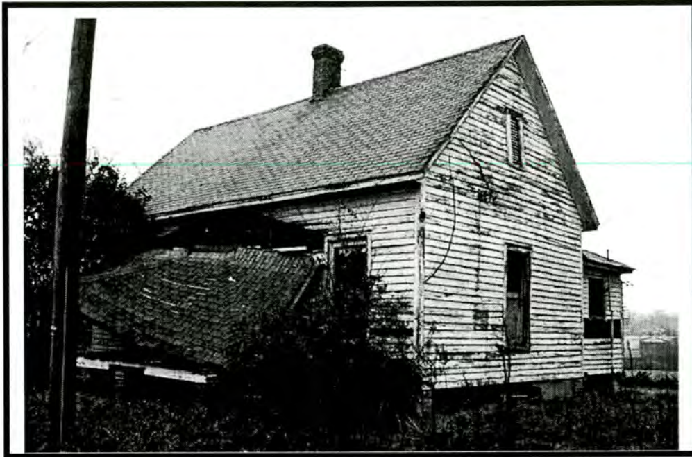
Figure 16 – Allen Street Mill Houses, House No. 3
