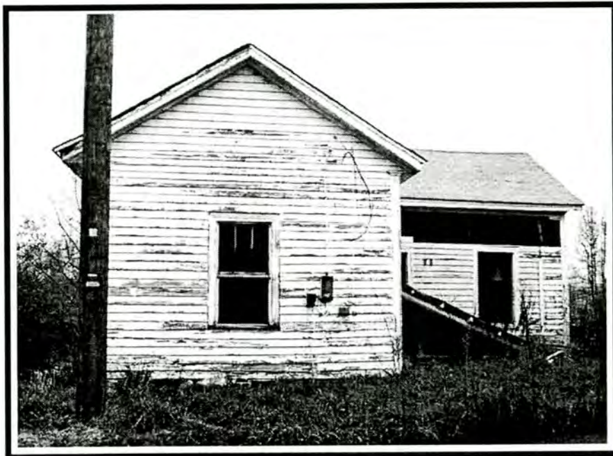
Figure 21 - Allen Street Mill Houses, House No. 8
