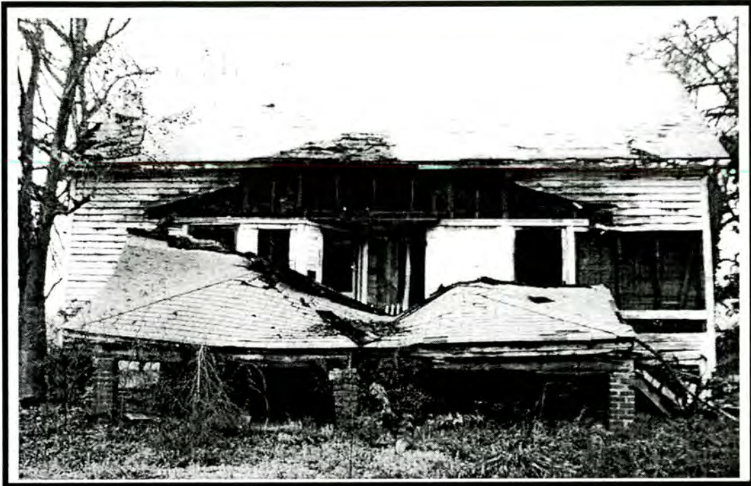
Figure 14 – Allen Street Mill Houses, House No. 1
