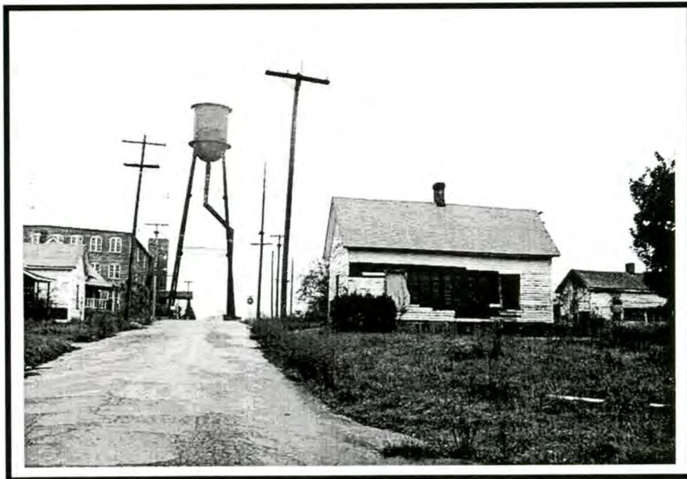
Figure 13 - Allen Street Mill Houses, looking East along Allen Street
