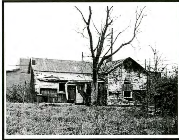
Figure 24 – Allen Street Mill Houses, House No. 11
