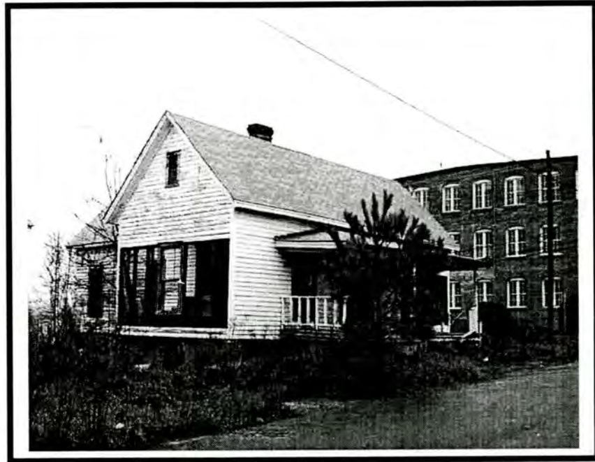
Figure 22 – Allen Street Mill Houses, House No. 9
