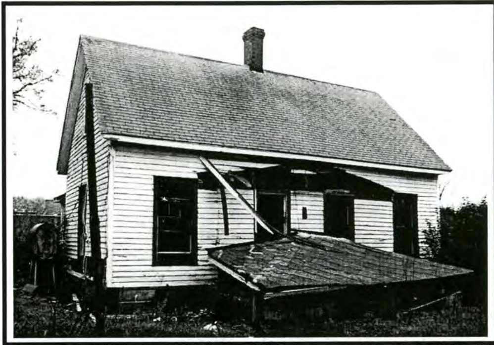
Figure 18 – Allen Street Mill Houses, House No. 5
