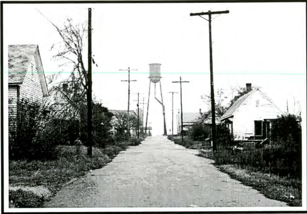
Figure 12 - Allen Street Mill Houses, looking East along Allen Street
