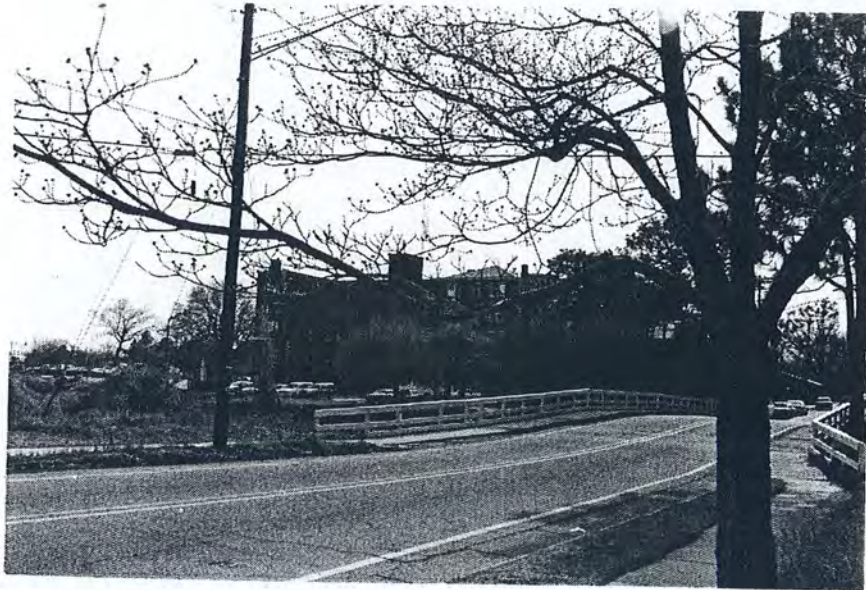
Plate 12. Setting, Hamlet Hospital Complex, Looking Southwest From Bridge.
