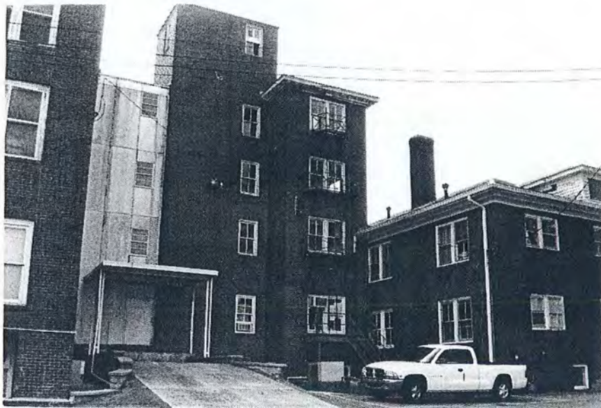
Plate 6. Hamlet Hospital, Rear (East) Elevation, Looking West.
