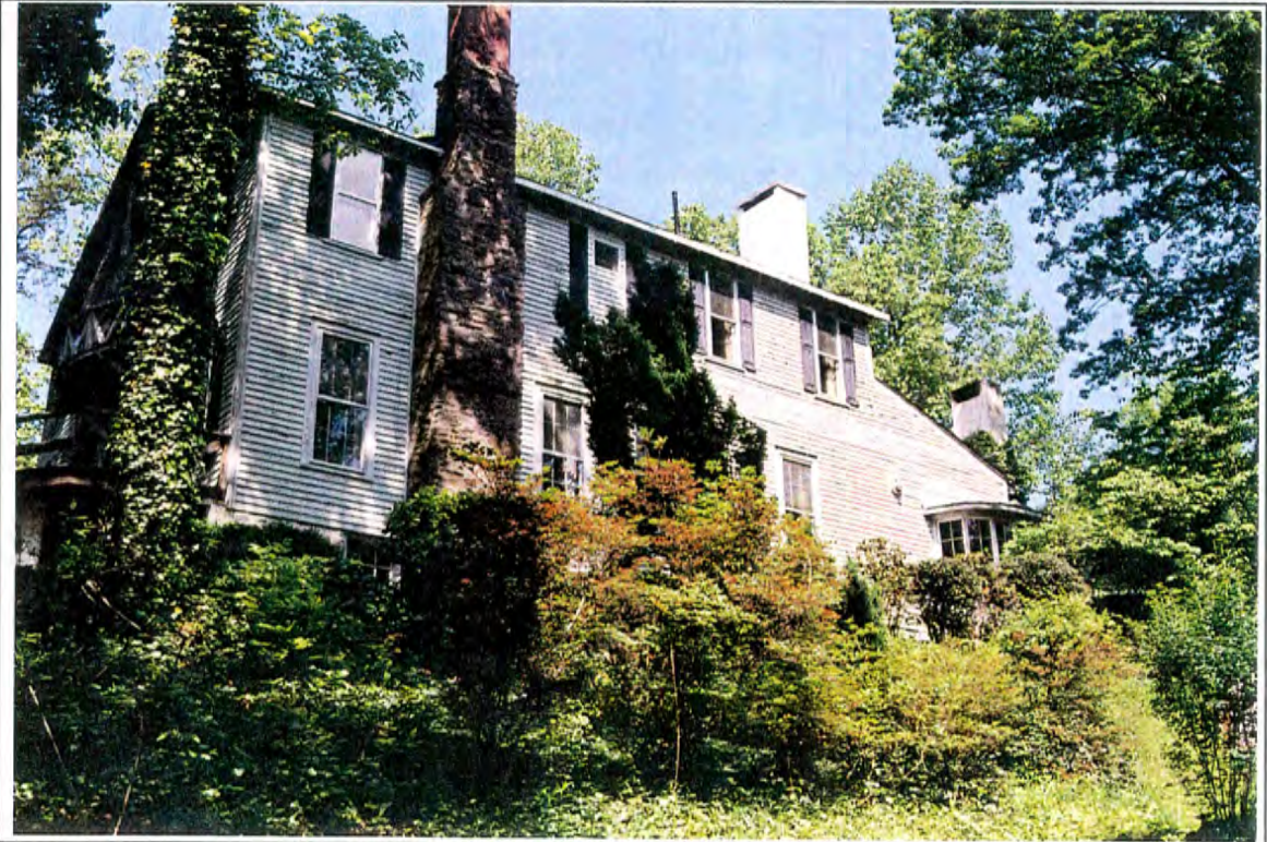
RIVER HOUSE, north elevation
