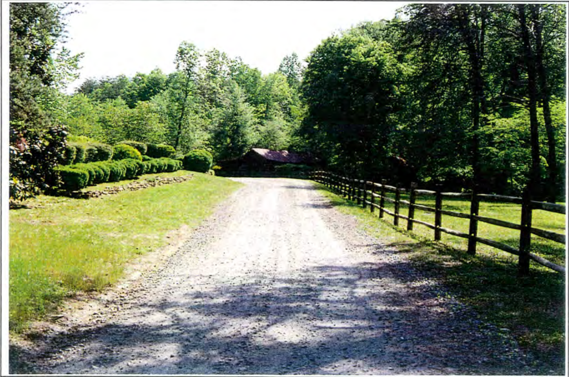
RIVER HOUSE, view to north along SR 1516
