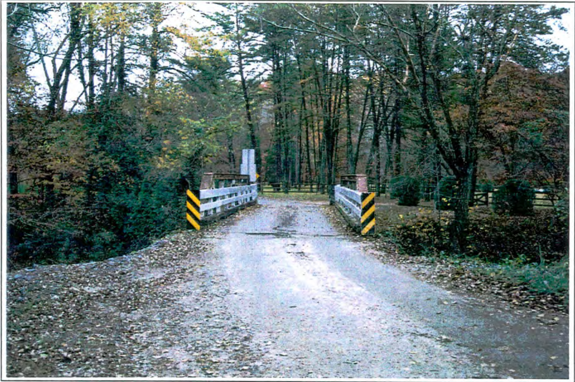
BRIDGE NO. 17 on SR 1516 over Pacolet River
