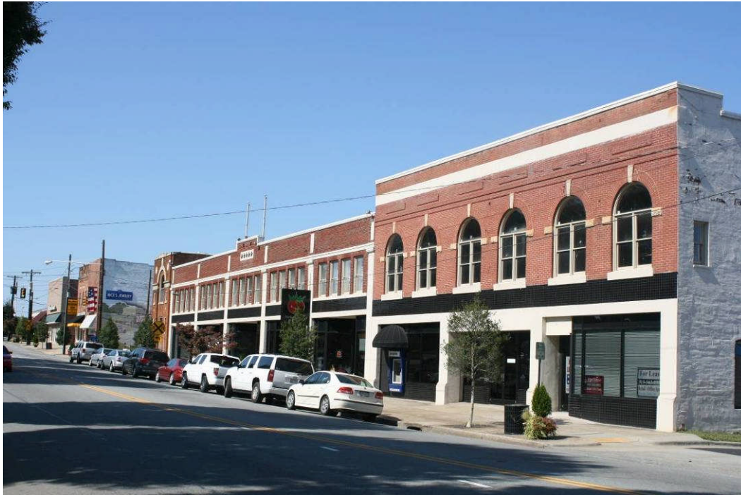
East Center Street, looking northwest
