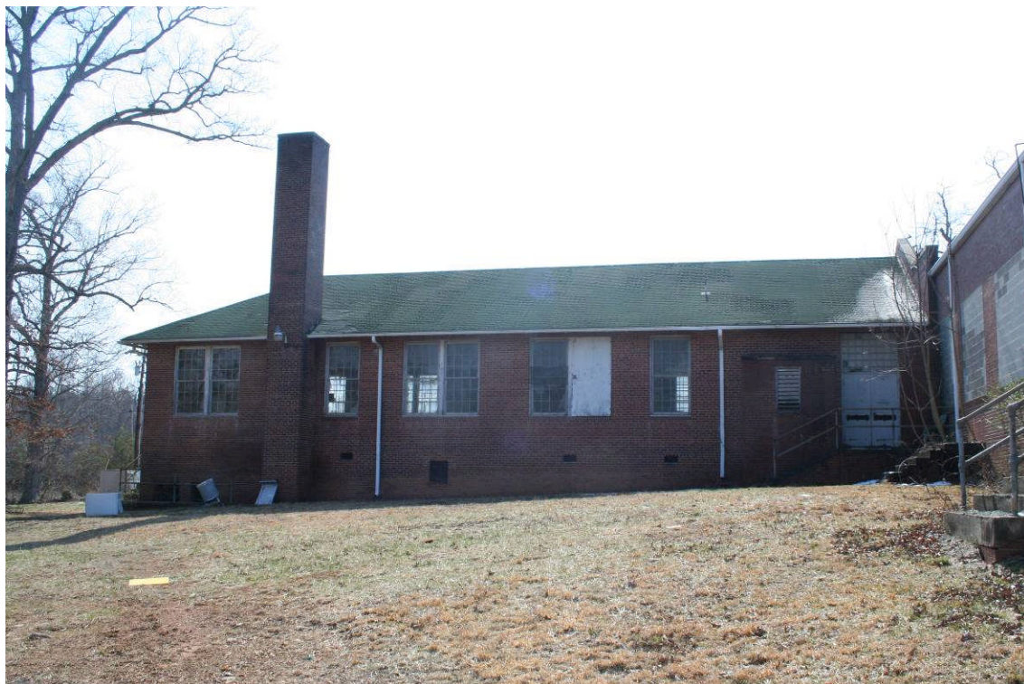
Rear auditorium wing
