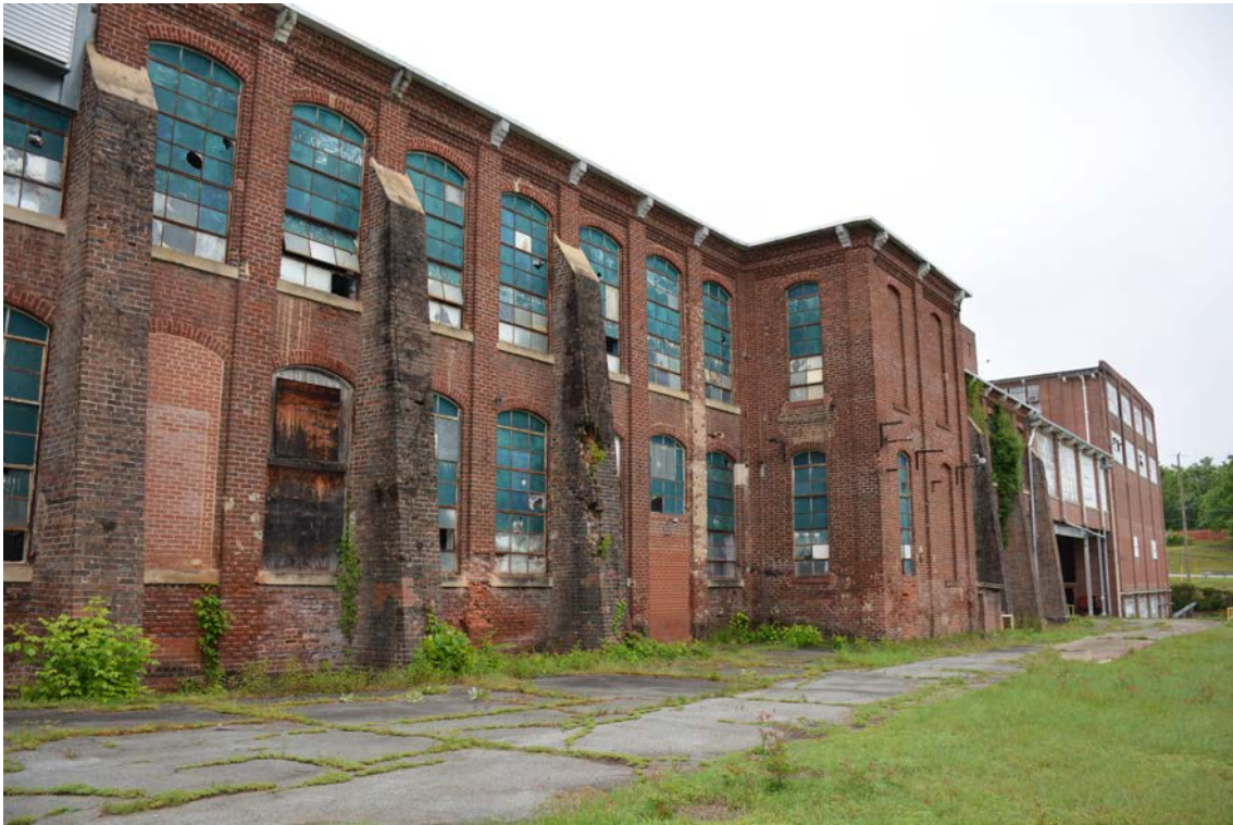
Building 15, west elevation, looking southeast
