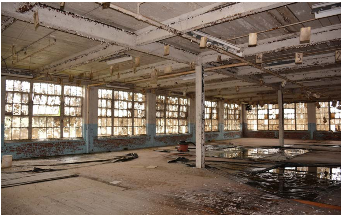
Building 16, Level 4, looking southwest
