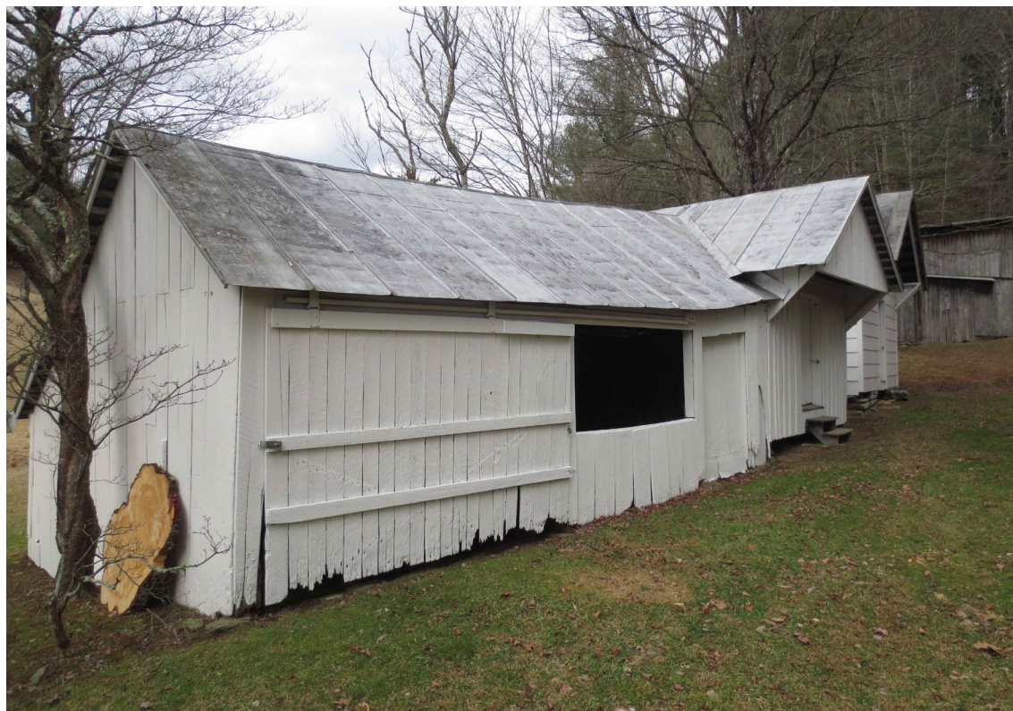
South and east elevations of carriage house/wood shop complex, looking north
