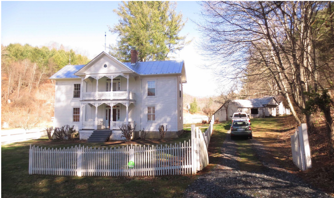
Front (south) elevation of main house, looking north
