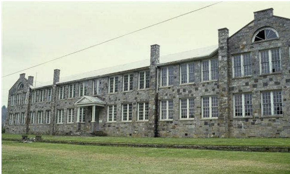
Façade of main school building
