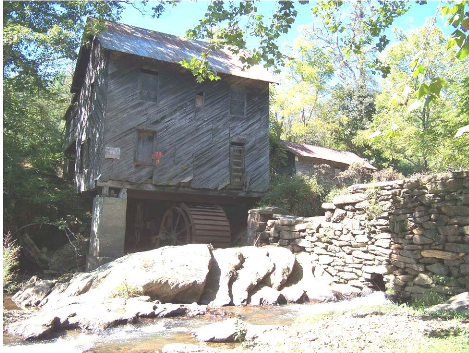
Dog Creek façade and dam view
